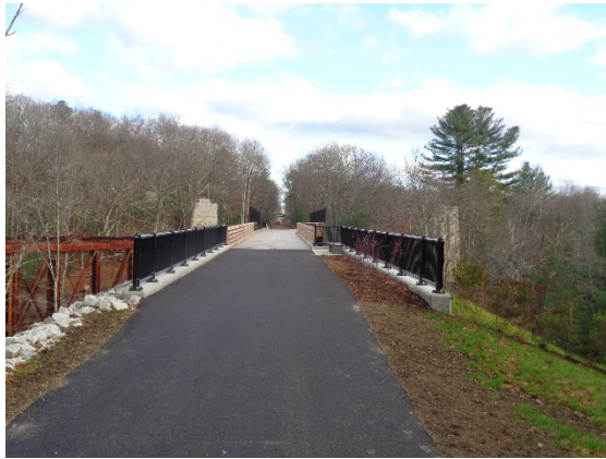
SNETT Bridge at Triad Bridges, Millville, MA
